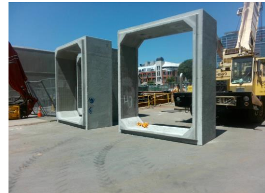
Reinforced Concrete Boxes for Storm Drain Relocation
