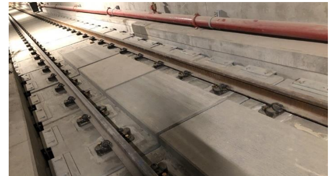
Direct Fastener plates and track assembled in left tunnel Reach 2
