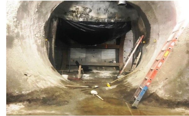
View of Reach 1 Cross Passage #8
