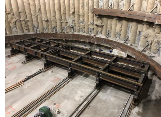
TBM Launch Cradle at Base of Excavated Tail Track Exit Shaft
