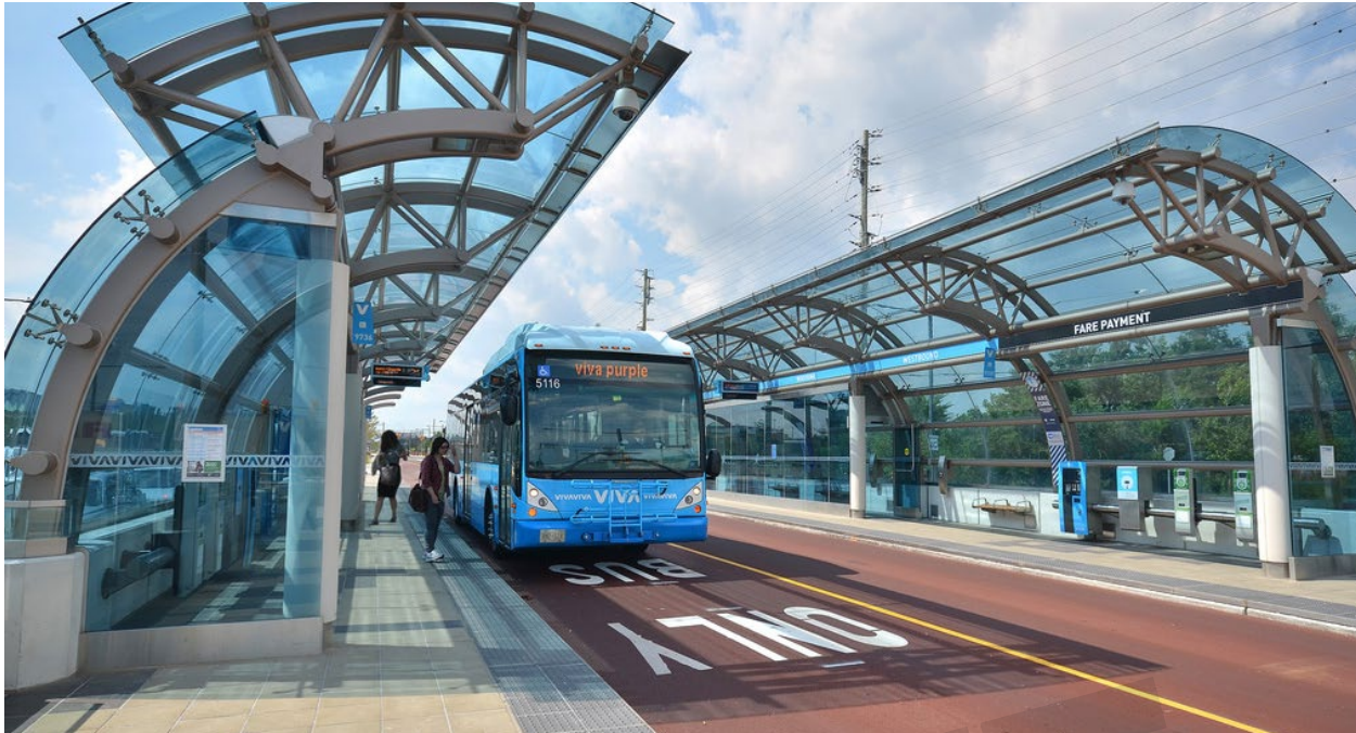
Access Control / Source: IBI Group
