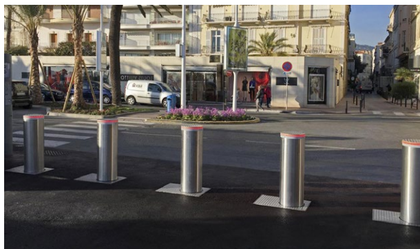
Current example of moveable bollards for access control / Photo Credit: National Signal
