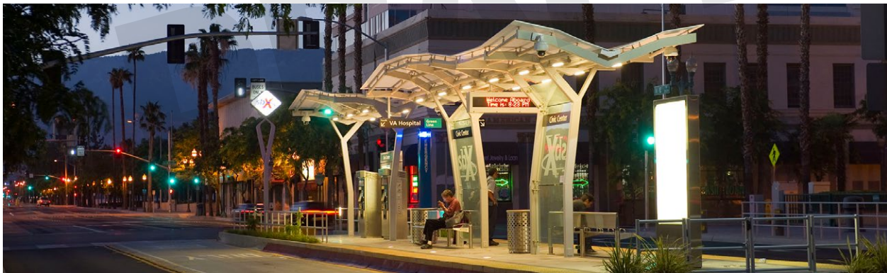
Lit canopy acts as beacon - Onmitrans SB, San Bernardino, CA Photo Credit: Gruen Associates
