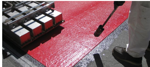
Thermoplastic Bus Lane Coating
