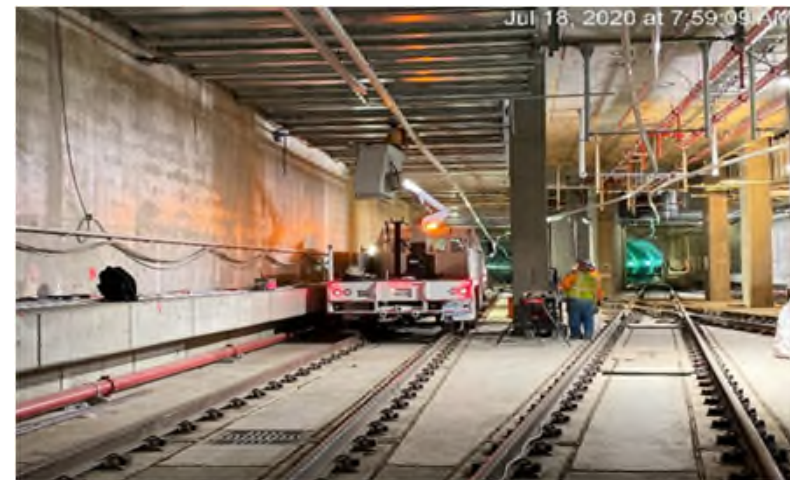
Continue installing supports and fixtures for the crossover lighting at the invert level of Expo/Crenshaw Station.
