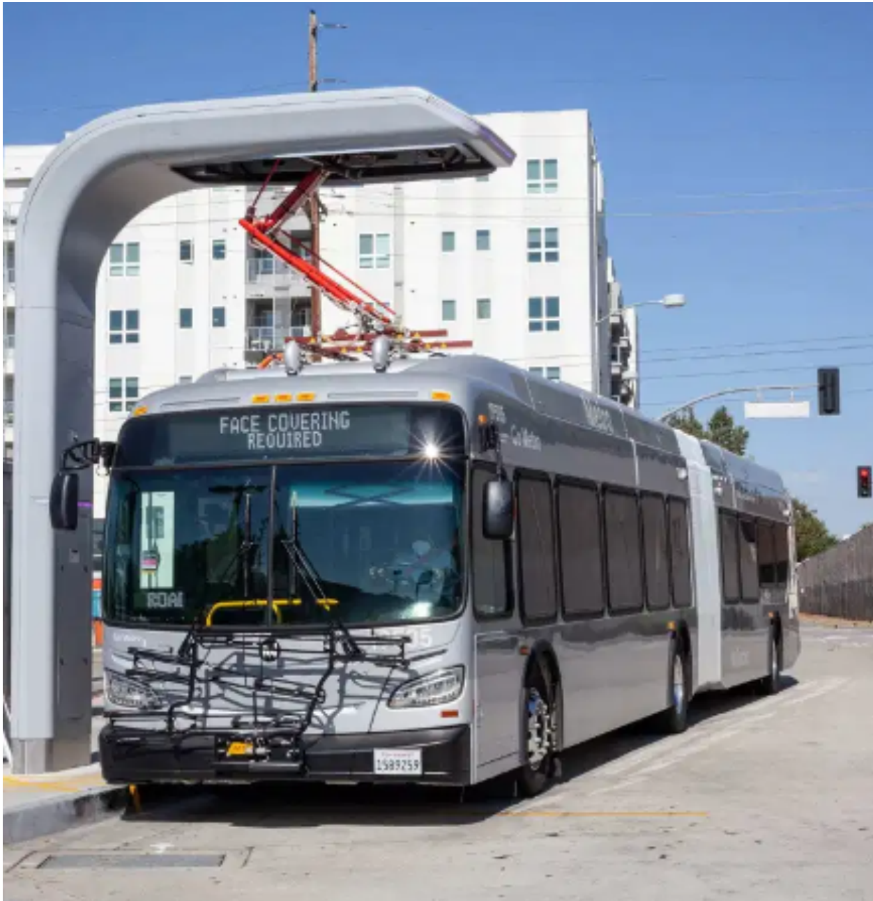
Figure 3-4. North Hollywood Station On-Route Charger
