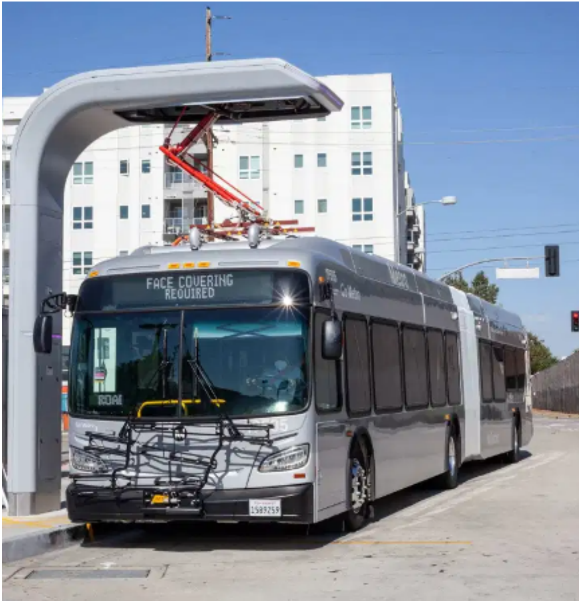
Figure E.2-1. North Hollywood Station On-Route Charger
