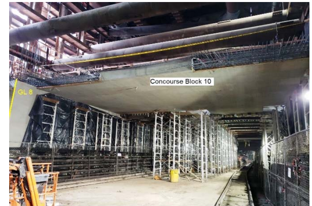
Wilshire/Fairfax Station Concourse Concrete
