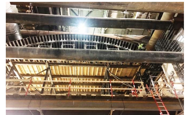
Roof Shoring Frames at Wilshire/La Cienega Station
