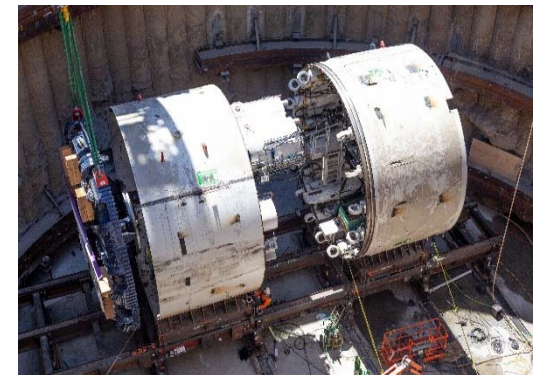
TBM Assembly at Base of Excavated Tail Track Exit Shaft
