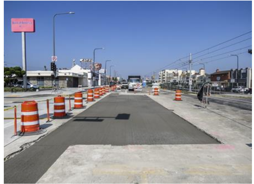
Crenshaw Street restoration at 57 th Street – looking southbound
