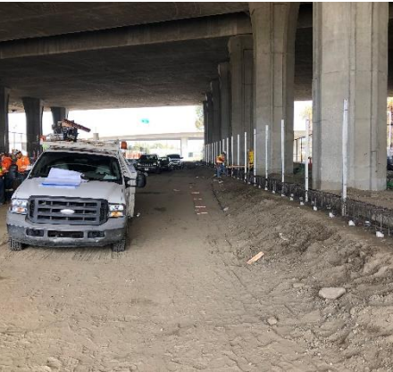
Grading Work @ Package B
