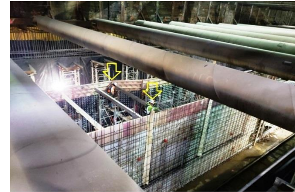
Wilshire/Fairfax Station Interior Wall Formwork
