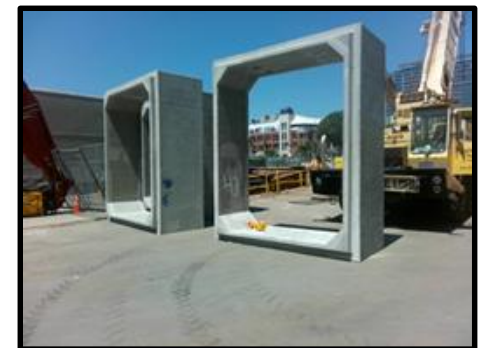
Reinforced concrete boxes for storm drain relocation.
