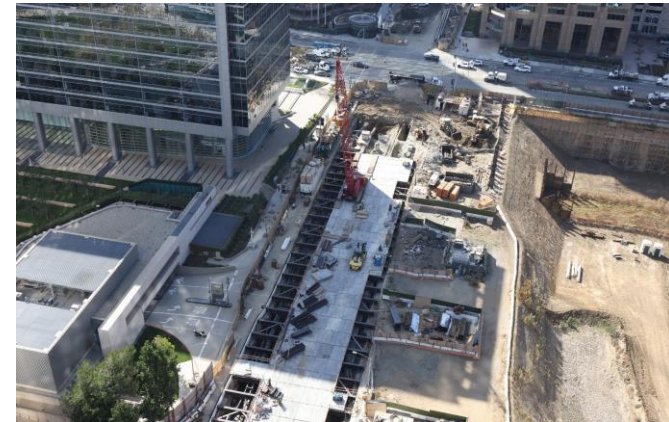
Piling and Decking Installation West of the TBM Launch Box
