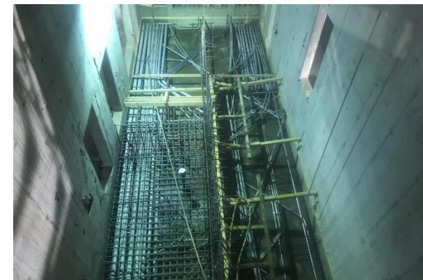
Track Level Conduit Installation at Wilshire/La Brea
