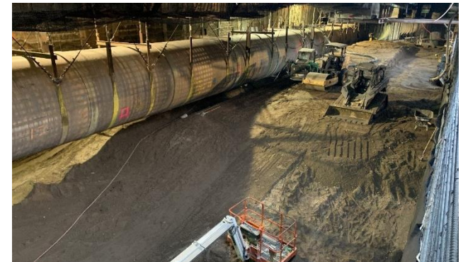
Backfill operations over station box at Historic Broadway Station
