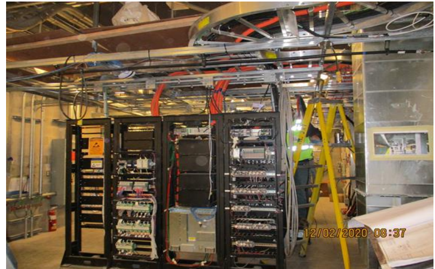
Leimert Park Station – contractor working on communication rack in train control and communication room.
