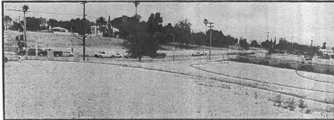
12. View of subject site, northwesterly facing from 1 st Street.
