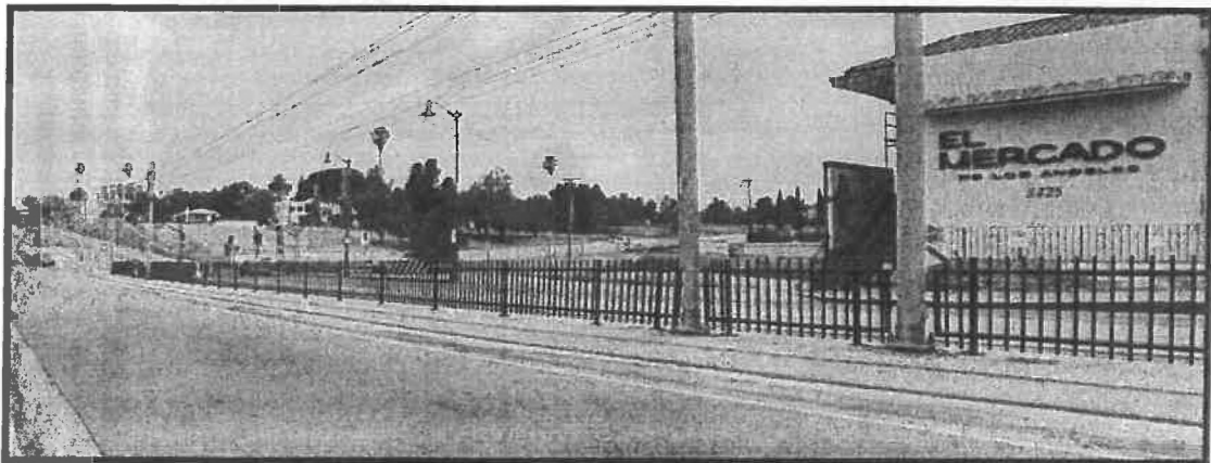
10. View of subject site, northwesterly facing from 1 st Street.
