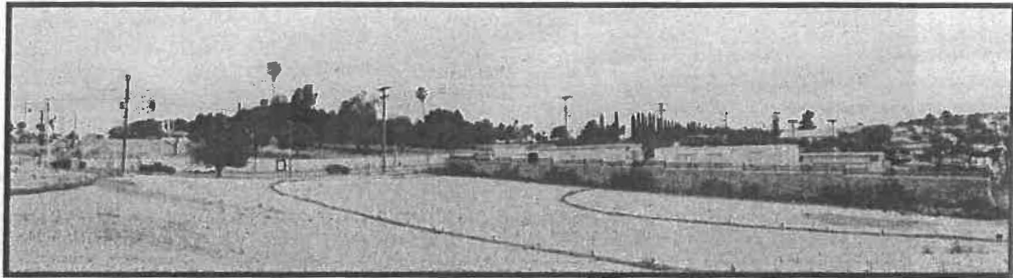
15. View of subject site, southwesterly facing from abutting alley.
