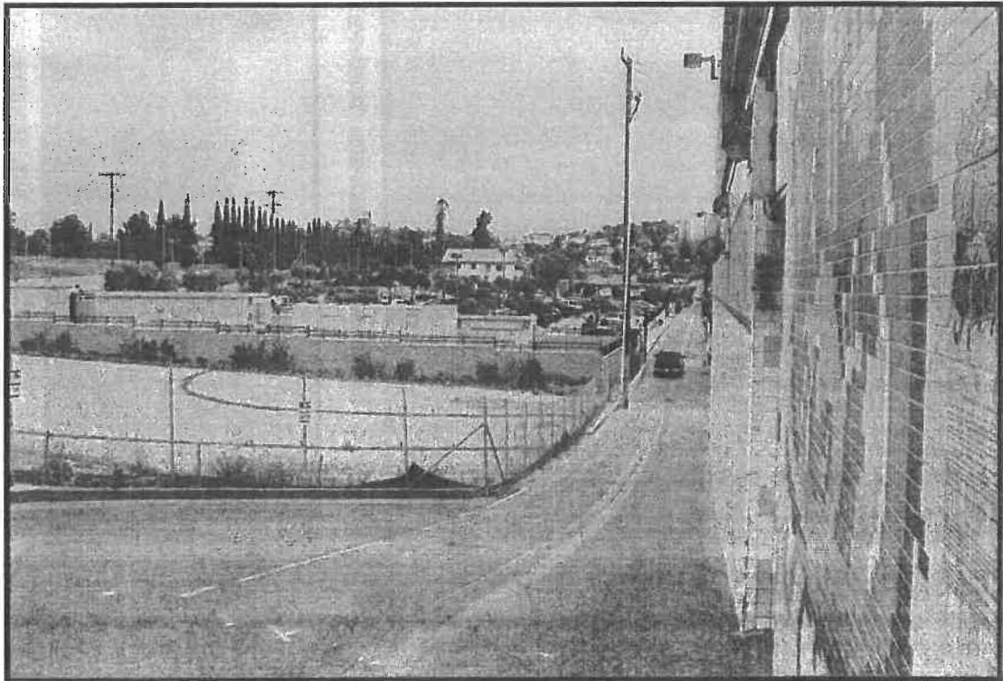
21. View of abutting alley, northeasterly facing from 1 st Street.
