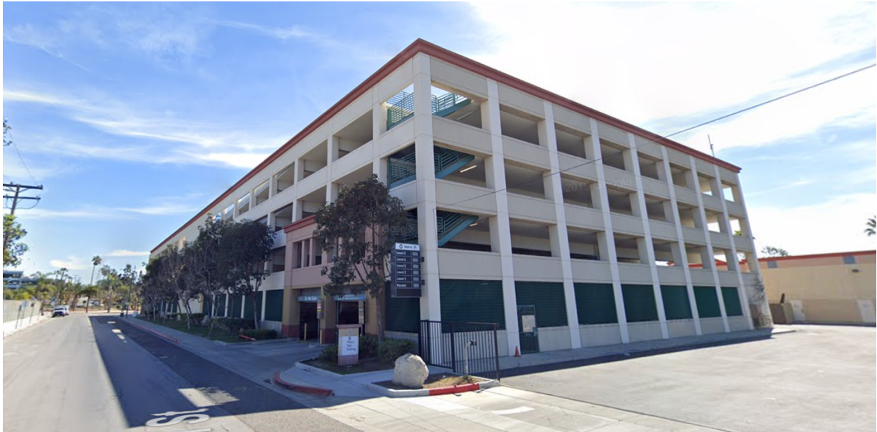
Figure 4.10.8 Willow Parking Garage (view from 27 th Street)
