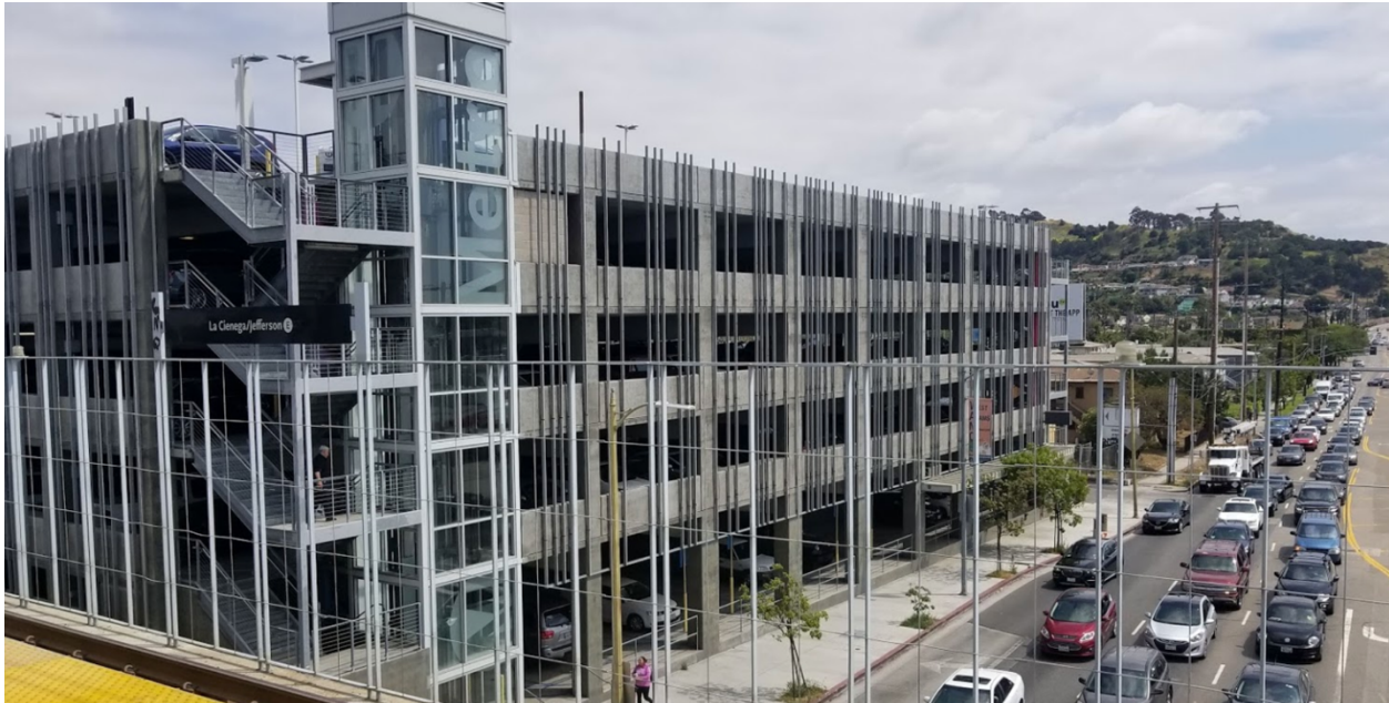
Figure 4.10.6 La Cienega/Jefferson Parking Garage (view from the station platform)
