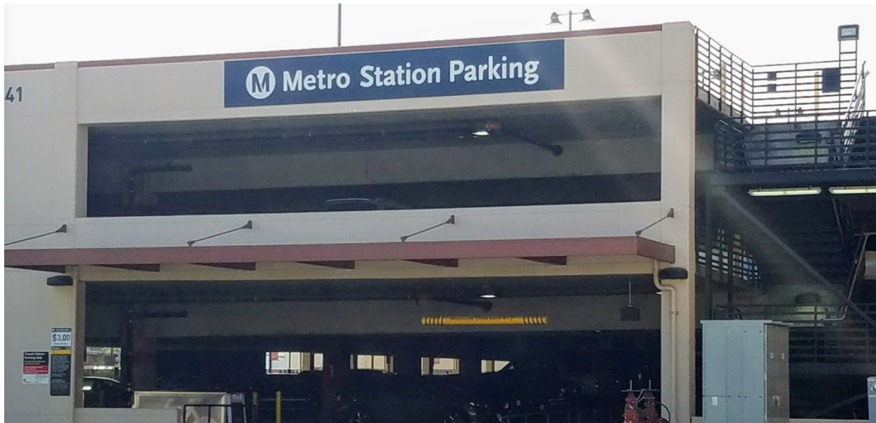
Figure 4.10.7 Monrovia Parking Garage (view from Primrose Avenue)
