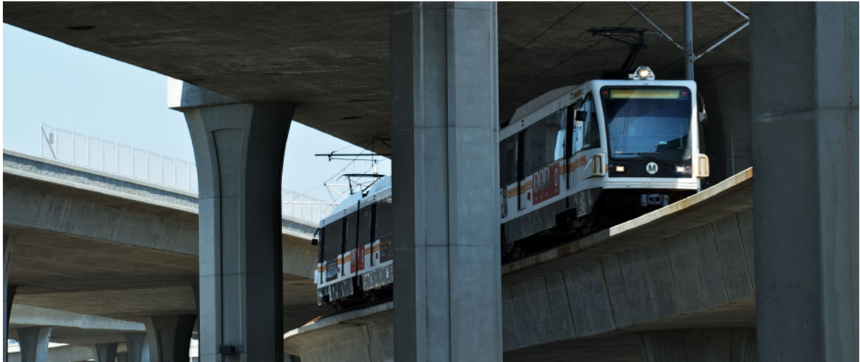
Figure 4.3.3 Metro C Line
