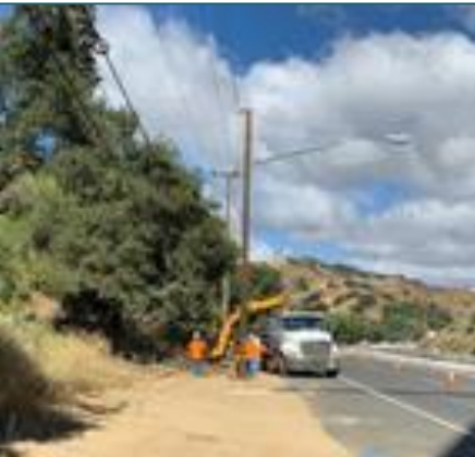
Old Road-SCE Power & AT&T Relocation
