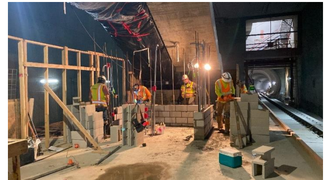
Conduit installation inside CMU Walls at Grand Av Art/Bunker Hill Station
