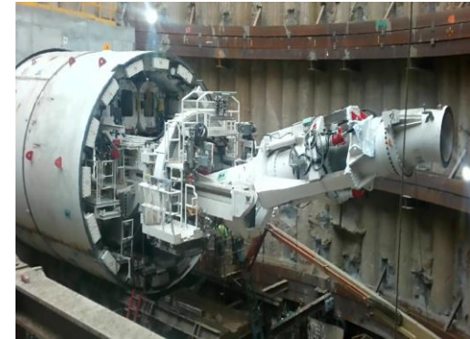
BL TBM Assembly at Tail Track Exit Shaft
