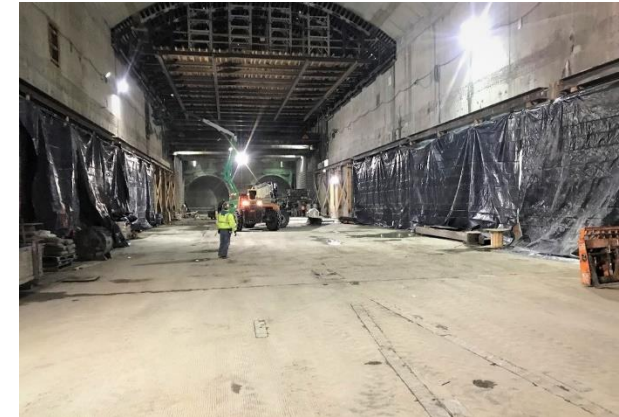
Track Level View of Wilshire/La Cienega Station
