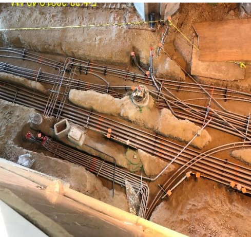
Underground utility work @ C Line west
