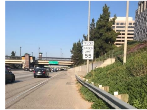
Newly Installed Speed Limit Sign
