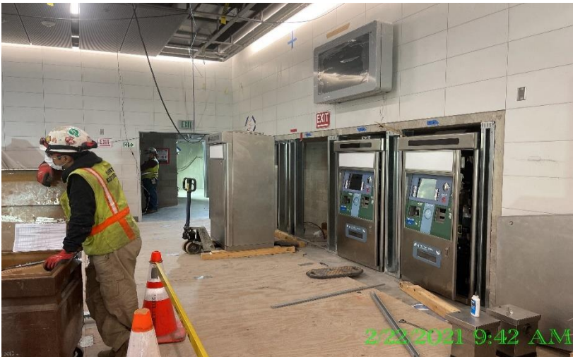
EXPO STATION – Installing and performing electrical work to the ticket vending machines at the Free Area.
