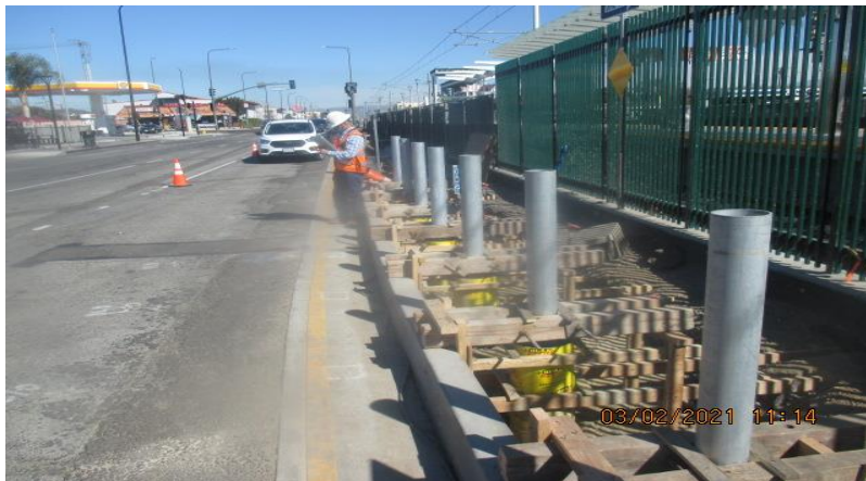
HYDE PARK STATION – Building formwork and installing bollards along the southbound median of the station.
