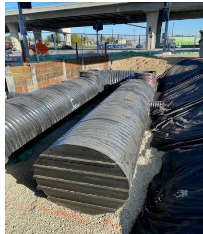
Installed cistern for North GSRD
