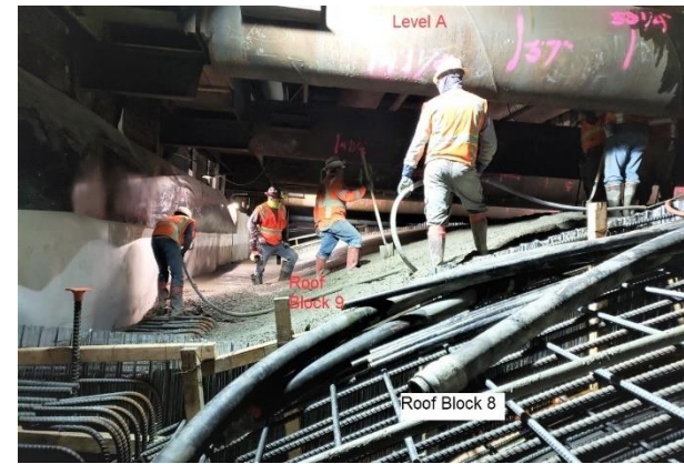
First Roof Concrete Placement at Wilshire/Fairfax Station
