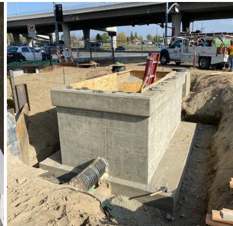
Formed & poured North Drainage System
