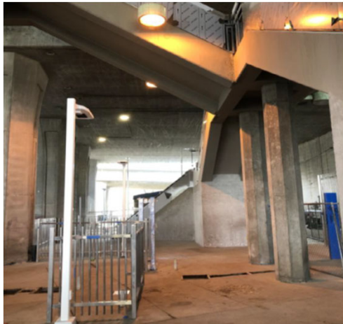
Completed concrete work @ C Line west
