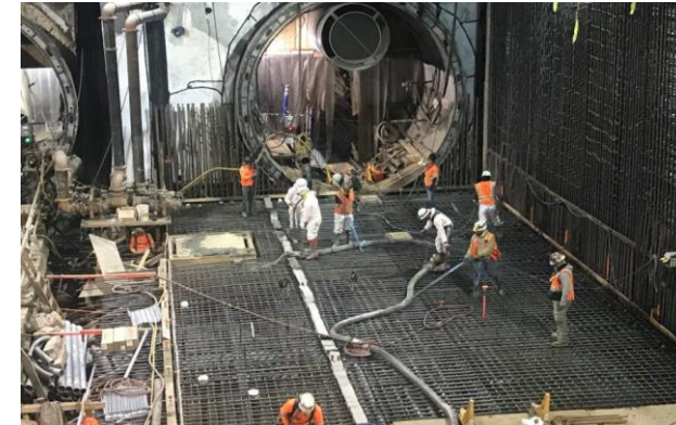
Wilshire/La Brea West Hammerhead Concrete Placement
