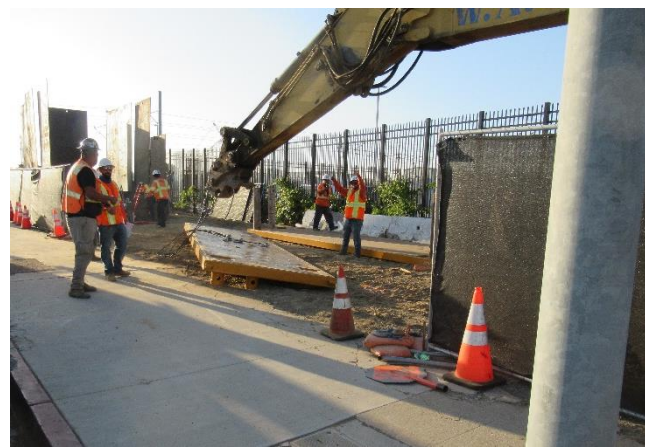
Duct Bank Work
