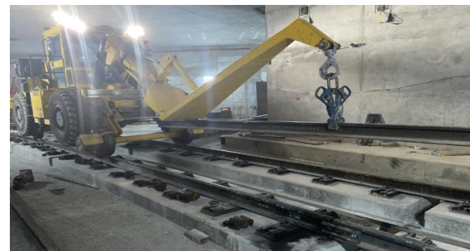
1 st Street Leg Plug Rail Installation
