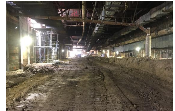
Constellation Station Box Excavation
