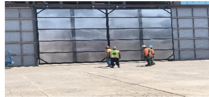
Gates Installed in Sound Wall at Construction Staging Area (UCLA Lot 36)
