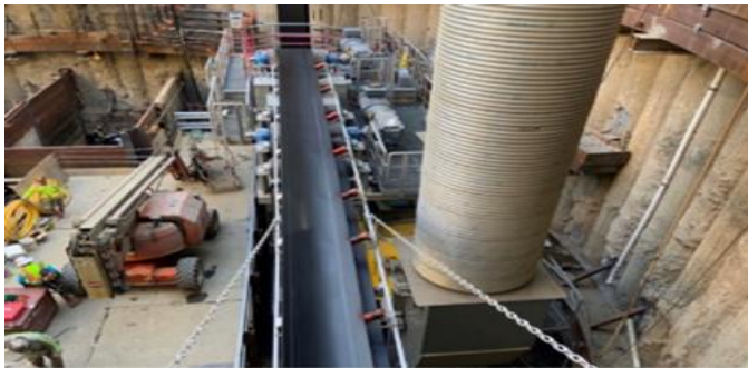
Conveyor Belt Tests at Tail Track Exit Shaft
