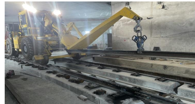
1st Street Leg Plug Rail Installation
