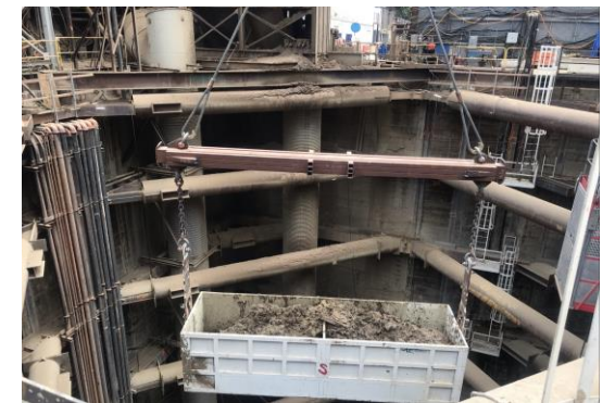
Tunnel Muck Removal in Century City
