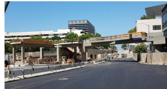
Asphalt pavement complete along Hope Street
