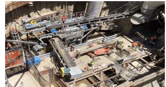
Muck Removal System at Bottom of Tail Track Exit Shaft
