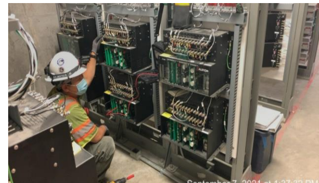
Train control testing at Flower T&C Room
