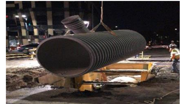
Sewer Relocation for Westwood/UCLA Station
