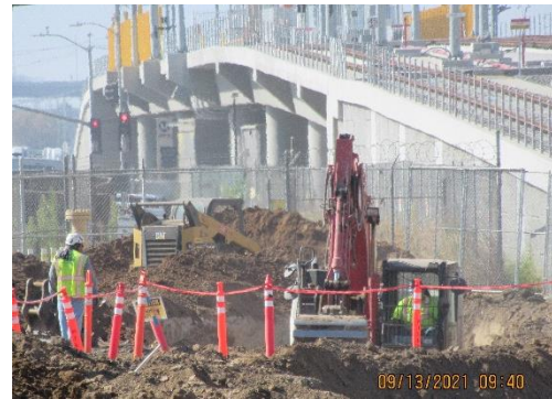
Backfill Work at South End of Site
