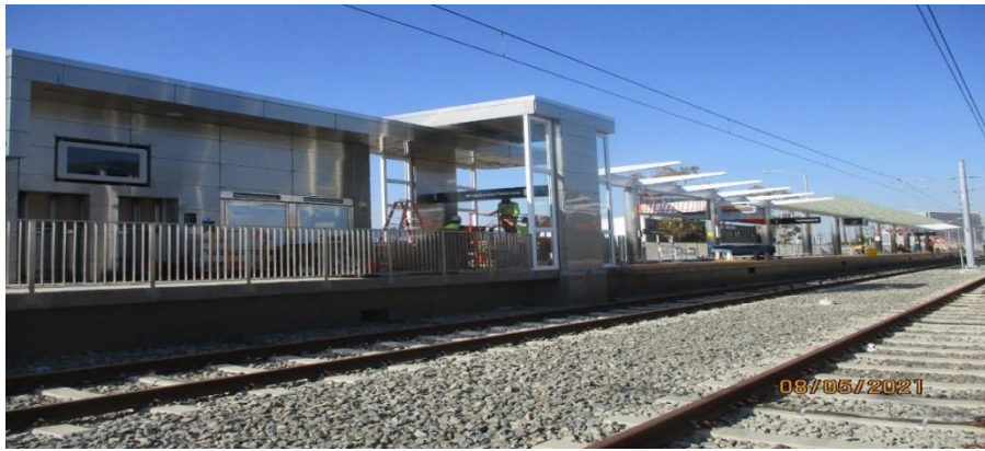
Hindry Station – Mounting wind screen glass
