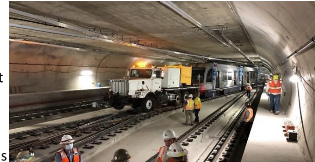
Dead pull test in Crossover Cavern
