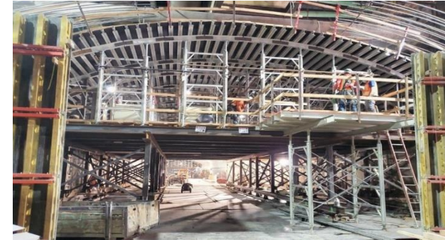
Roof Falsework Installation at Wilshire/Fairfax Station
