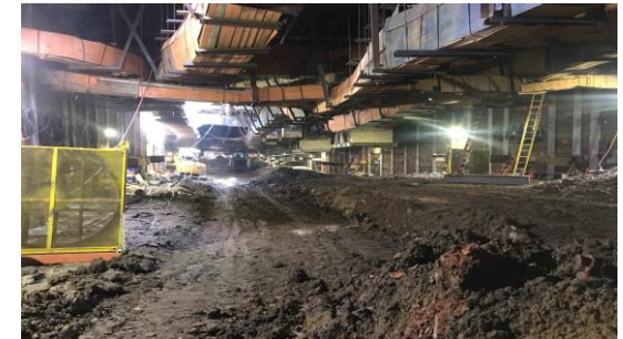
Constellation Station Box Excavation
