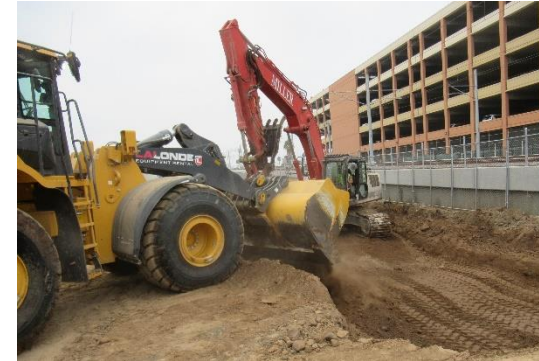
On Site Backfilling Work
