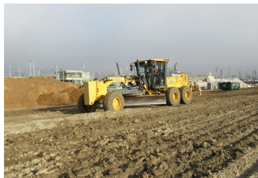
Backfill Work at South End of Site
