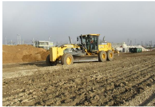
Backfill Work at South End of Site
