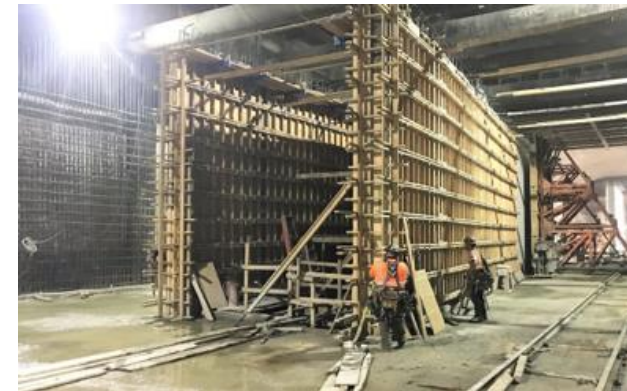
East Interior Wall Formwork at Wilshire/La Cienega
