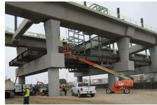
LAVA APM Steel Work in Progress
