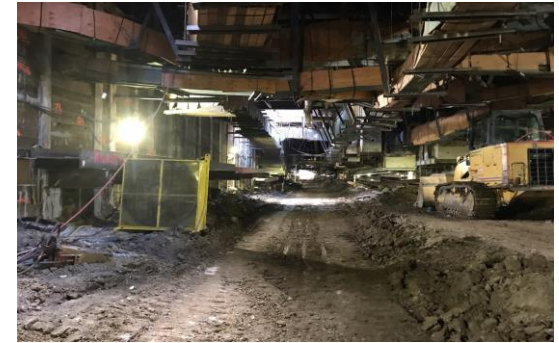
Constellation Station Box Excavation
