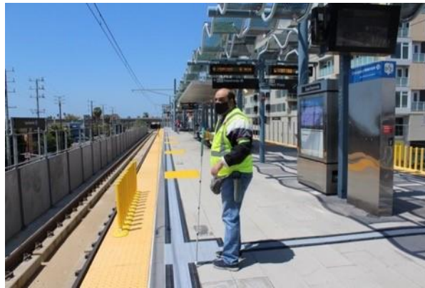
Figure 19: Tactile Paths on the E (Expo) Line Platform
