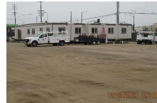
Mobilization for Main Station Construction
