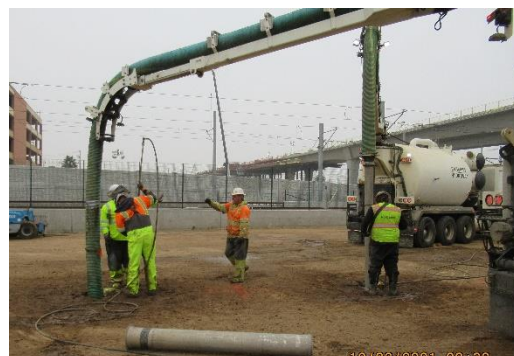
Potholing for Stormwater Capture System
