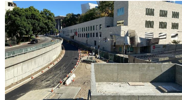
Concrete curb & gutter at 2nd Place/Flower
