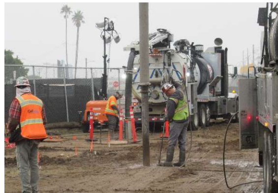
Shoring installation for Stormwater System
