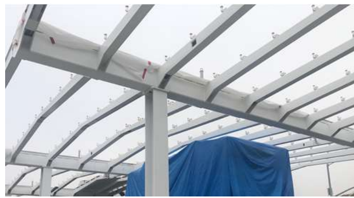
Little Tokyo/Arts District Station Canopy Installation
