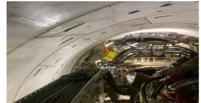
Ring Installation in the BL Tunnel
