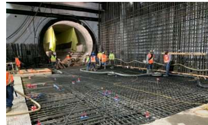
Concrete Placement at Wilshire/La Cienega Station (West)
