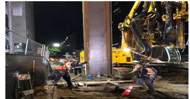
SOE Pile Installation Along North Side Wilshire Blvd.
