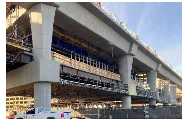
LAWA Station work in progress
