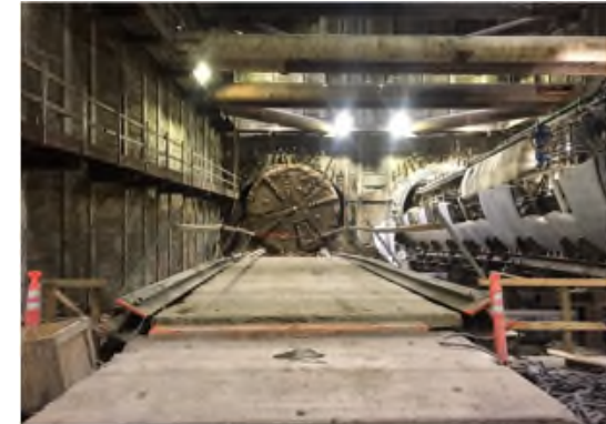
Ruth Breakthrough at Wilshire/Rodeo Station
