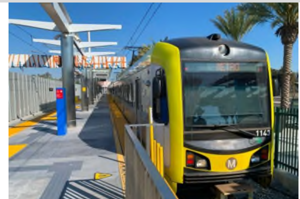
Downtown Inglewood Station – Train testing
