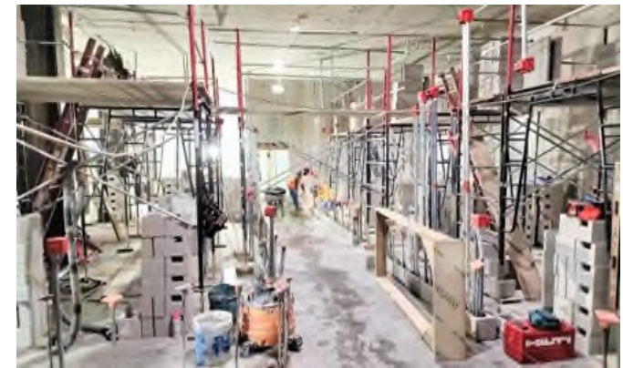
CMU Block Wall Installation at Wilshire/Fairfax Station
