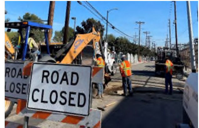
DWP Sylmar Undergrounding
