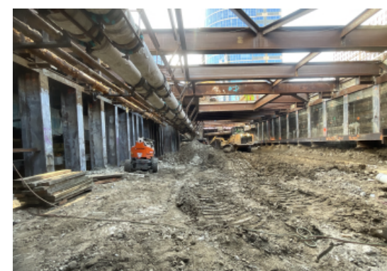
Constellation Station Entrance Excavation
