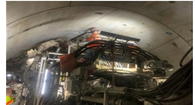
Ring Installation in the BL Tunnel
