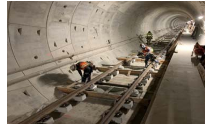
Reach 1 North Tunnel Trackwork Installation
