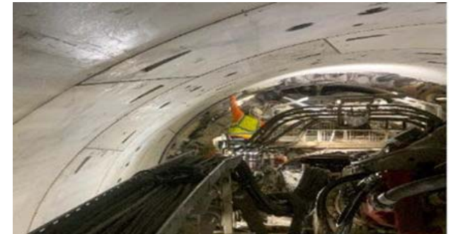
Ring Installation in the BL Tunnel
