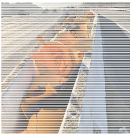
Damaged crash cushion from accident during holidays
