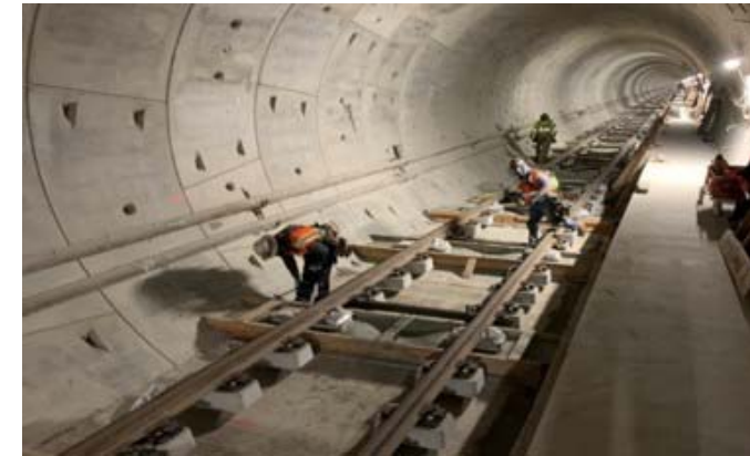
Reach 1 North Tunnel Trackwork Installation
