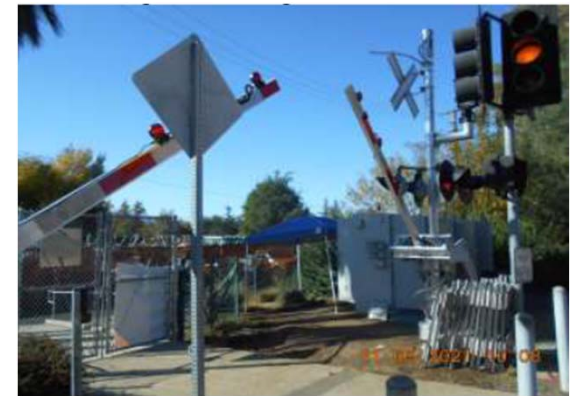
Pilot Gate - Testing
