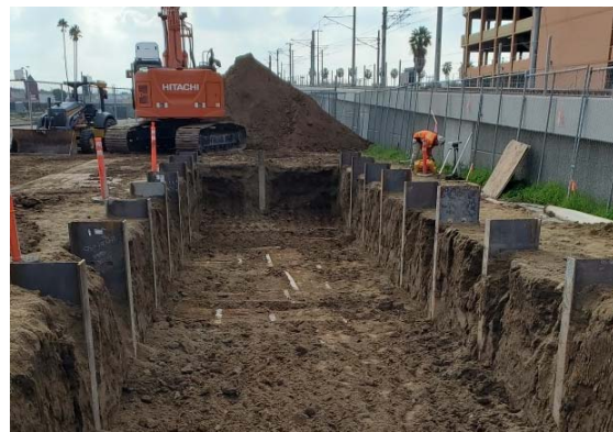
Shoring in progress
