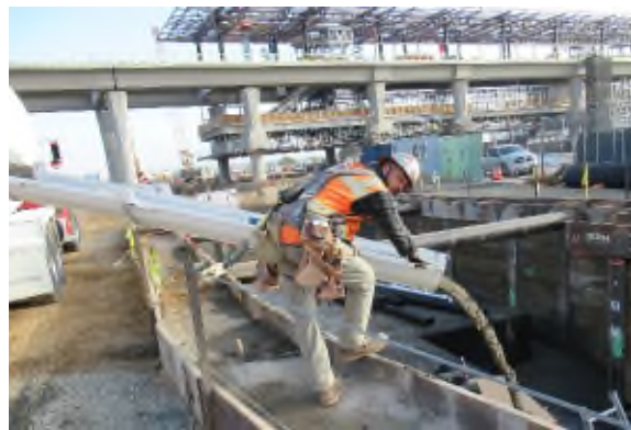
Backfill at cisterns
