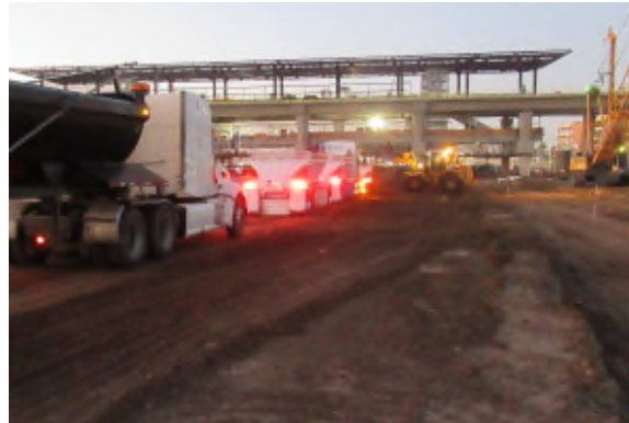
Early morning soil removal work
