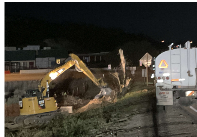
I-5-SB / Cal-Grove Blvd on-ramp clearing and grubbing work in progress
