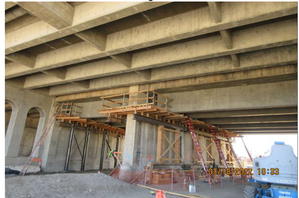
1 st Bridge – Bent 16
