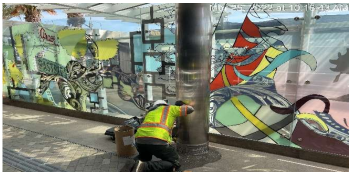
Hyde Park Station – Applying anti-graffiti shield
