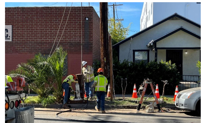
DWP Vesper Advanced Utility Relocation
