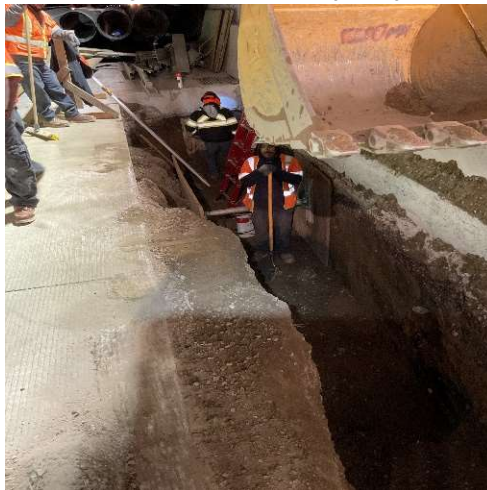
Drainage excavation on SB I-5 median DS# 159
