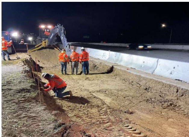
Roadway excavation Stage 1 Phase 1 on SB Pico/Lyons RT shoulder
