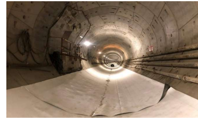
Layout HDPE in Reach 2 Tunnel
