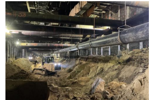
Century City Constellation Station Box Excavation
