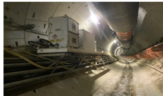
BL Tunnel Booster Fan & Transformer Installation
