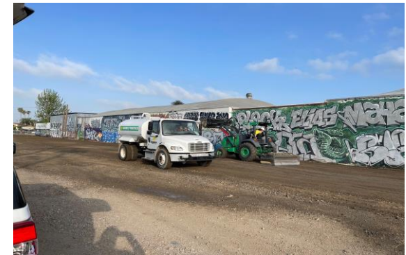
Site preparation work
