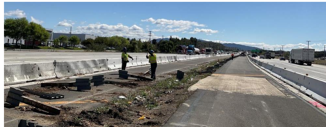
Removal of existing metal beam guardrail from median – Rye Canyon Road to Parker Road
