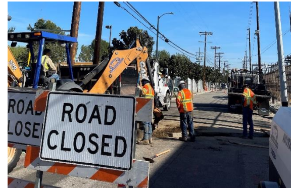
DWP Sylmar Undergrounding
