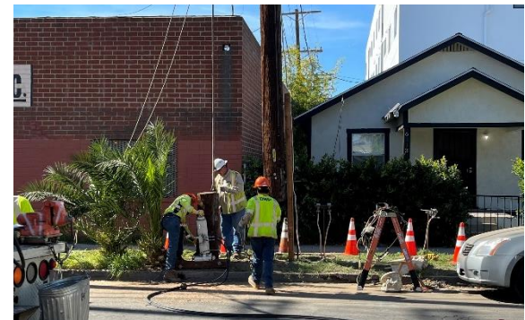
DWP Vesper Advanced Utility Relocation
