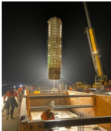
Erection of Column for new Weldon Canyon bridge
