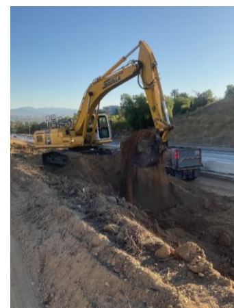
Median Excavation work for retaining walls in progress
