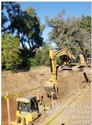
Excavation for DS 11-7 (RCB) – SB71
