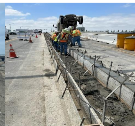
Valley View median construction
