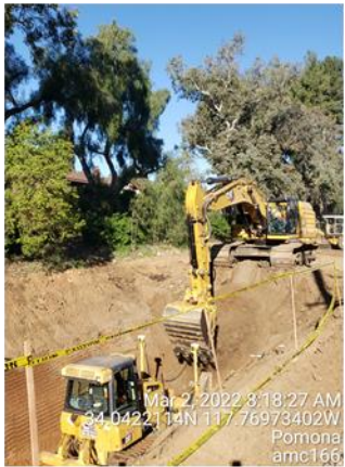
Excavation for DS 11-7 (RCB) – SB71
