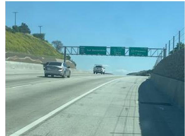
Overhead sign structure at Kellogg Hill
