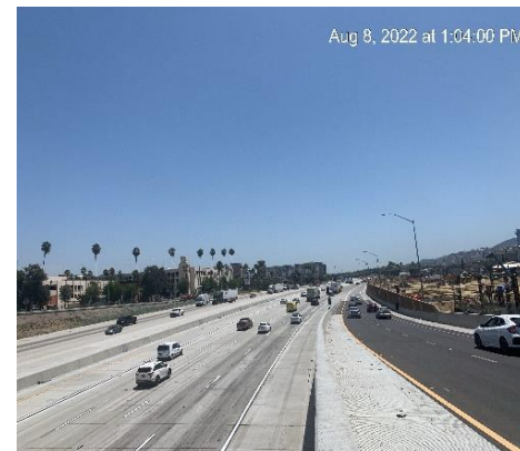
SB RTE. 5 MAINLINES OPENED TO TRAFFIC – MAINLINE FINAL STRIPING COMPLETED: (LEFT) SB RTE. 5 BURBANK BLVD. ONRAMP / (RIGHT) SB RTE. 5 MAINLINE AT BURBANK BLVD. OVERCROSSING
