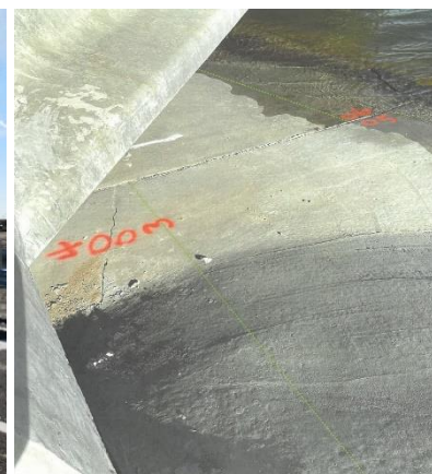
Channel Lining Cracks
