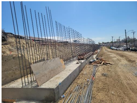
RW 815 – SB 405 Crenshaw Blvd off ramp widening – Looking South
