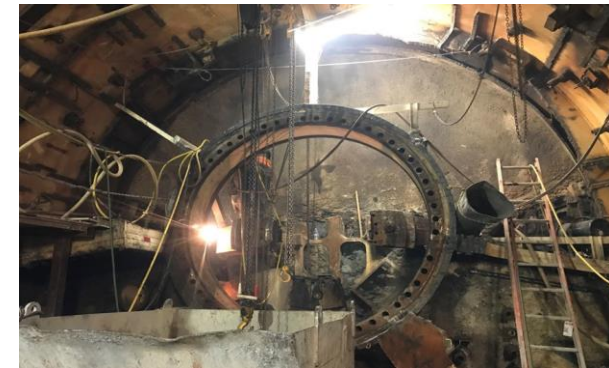
North Tunnel TBM Cutterhead Removal
