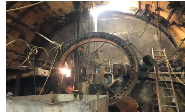
North Tunnel TBM Cutterhead Removal
