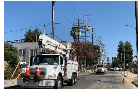
DWP Overhead Construction at Vesper
