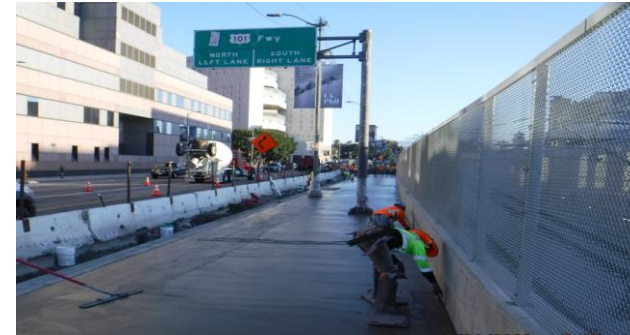
Concrete pour for 1st Street sidewalk (Temple & Commercial)
