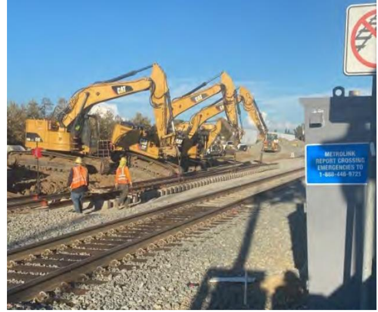
Garey East – Metrolink Turnout installed
