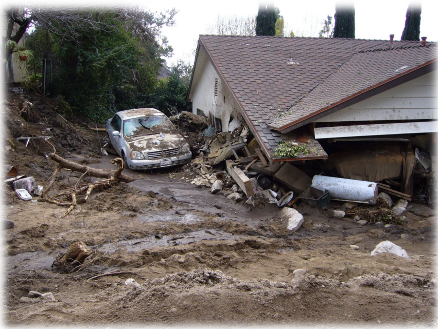
Caption: House damaged by debris flows generated in Mullally Canyon in response to a rainstorm on February 6, 2010. The drainage basin above this home was burned the previous summer by the Station Fire, which was the largest fire in the history of Los Angeles County at the time.
