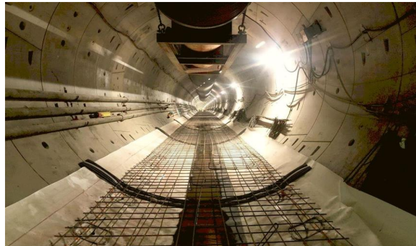
Reach 3 Tunnel (Fairfax to La Cienega) Tunnel Invert Construction
