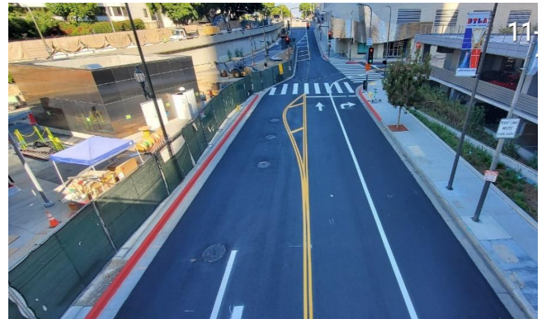
Final asphalt concrete paving along Hope St
