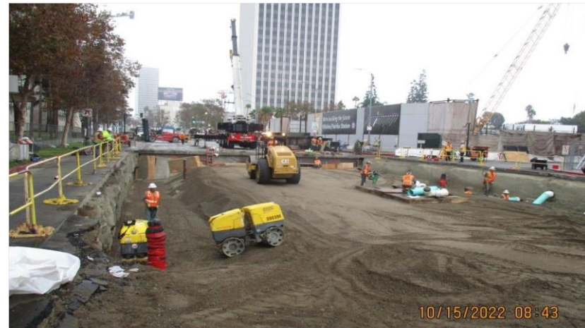
Wilshire/Fairfax Weekend Street Restoration Work
