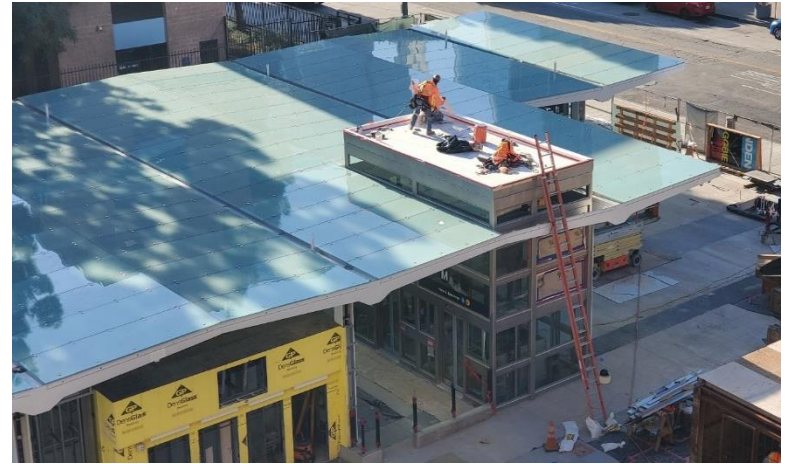
Installation of TPO roofing (Historic Broadway Station)
