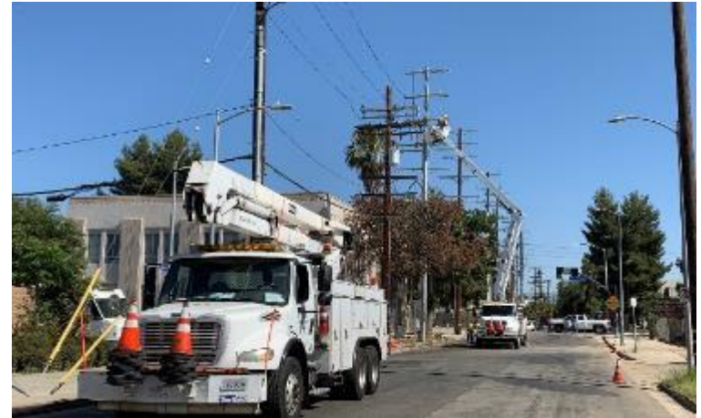
DWP Overhead Construction at Vesper
