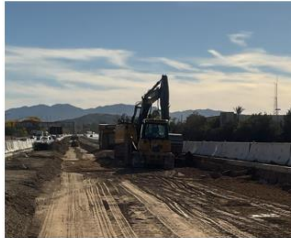
On-Going Roadway Excavation in the Median
