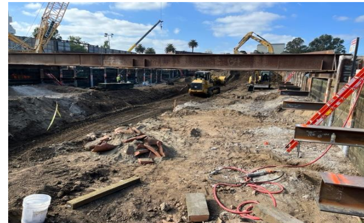
Westwood/VA Station: Excavating station to Level 1 Bracing
