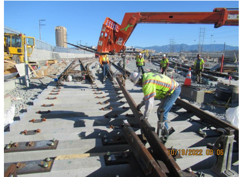
North Yard Storage Tracks
