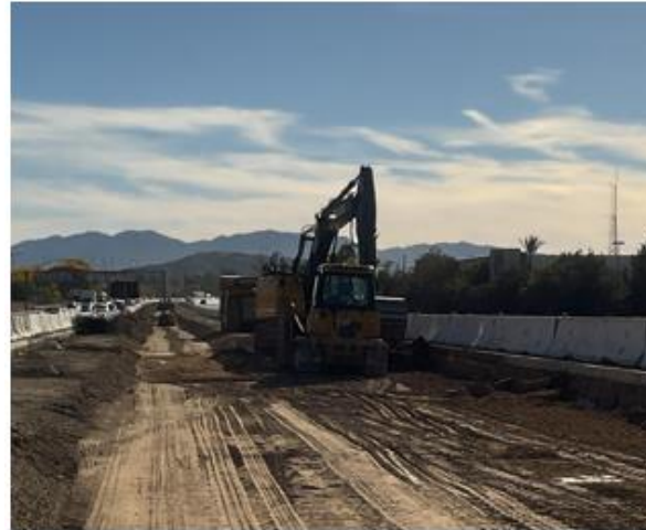
On-Going Roadway Excavation in the Median
