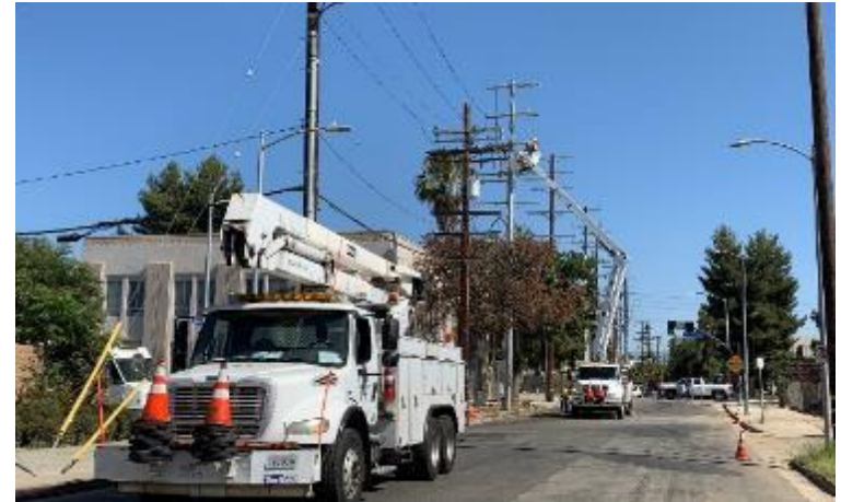
DWP Overhead Construction at Vesper
