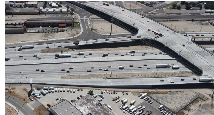
I-5 South/Carmenita Interchange
