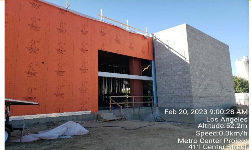
Exterior Finish – Weather Barrier & Sheet Metal
