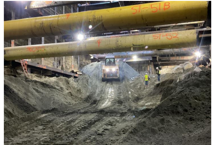
Century City Constellation Station - Excavation Progress
