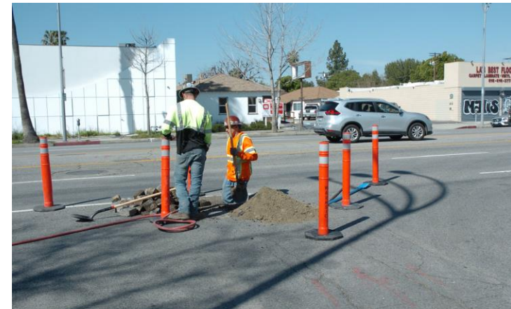
W.A. Rasic crew performing potholing on Van Nuys Blvd.
