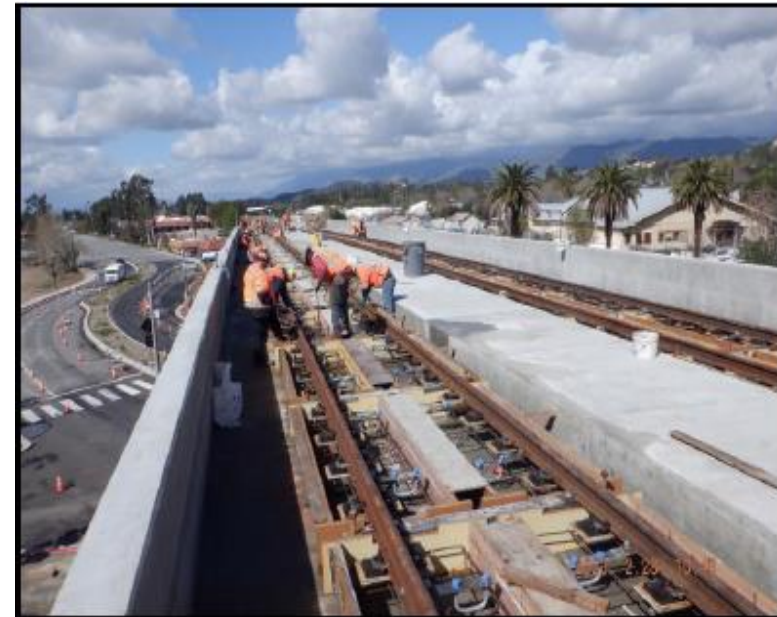
Bonita / Cataract – Structure Track Direct fixation
