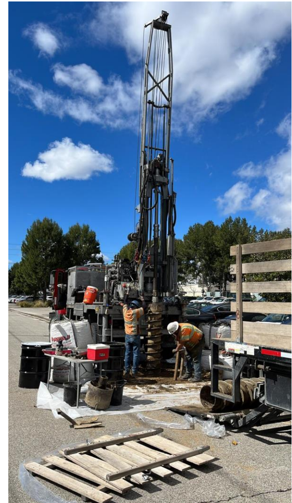
Geotech- percolation testing for stormwater capture scope
