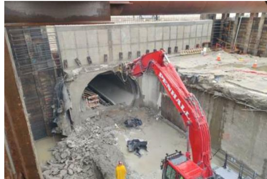
West Portal Wall Demolition
