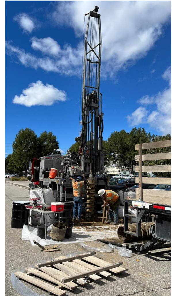
Geotech- percolation testing for stormwater capture scope
