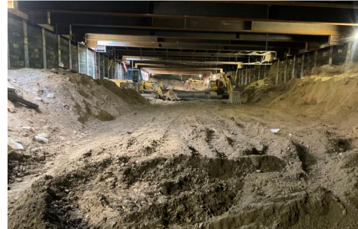
Westwood/UCLA Station: Excavation underneath Wilshire Blvd
