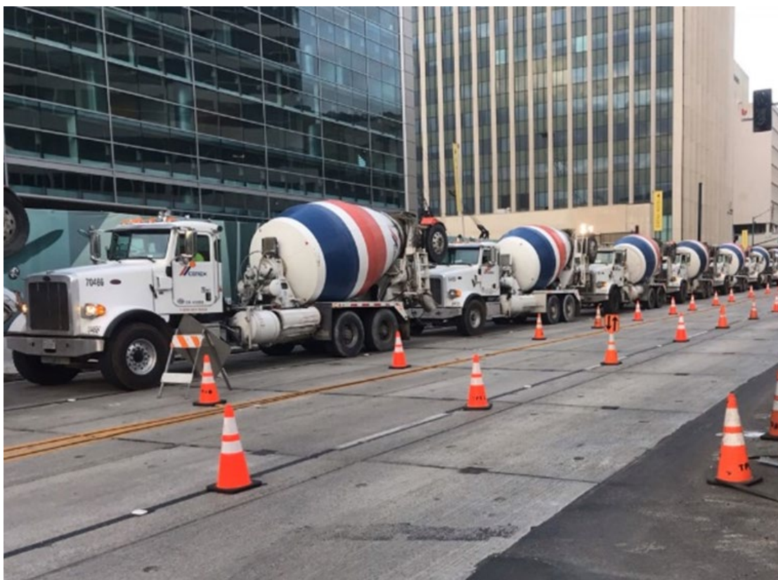
Concrete trucks on Wilshire Blvd awaiting delivery to Rodeo station for concrete slab
