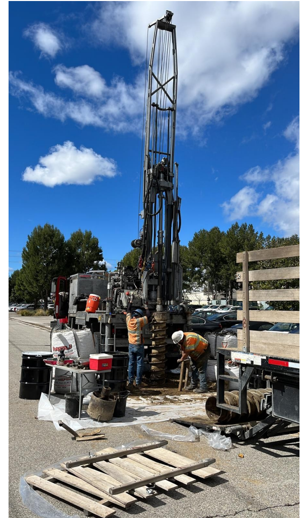
Geotech- percolation testing for stormwater capture scope
