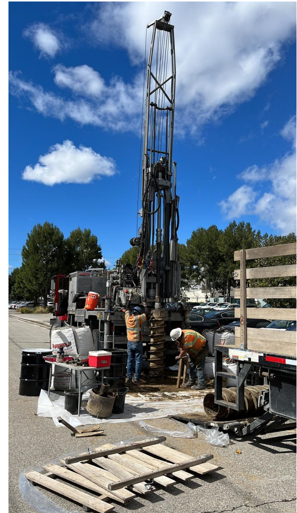
Geotech- percolation testing for stormwater capture scope
