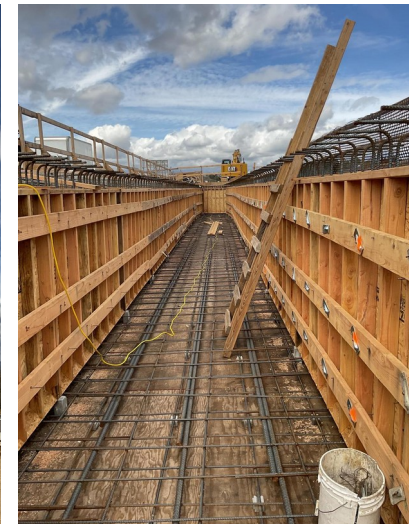
Carpentry work at Butte Canyon Bridge
