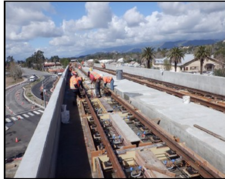
Bonita / Cataract – Structure Track Direct fixation
