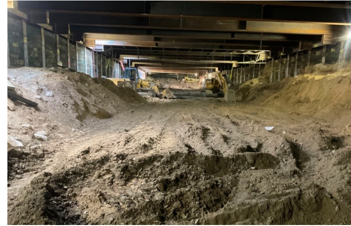
Westwood/UCLA Station: Excavation underneath Wilshire Blvd
