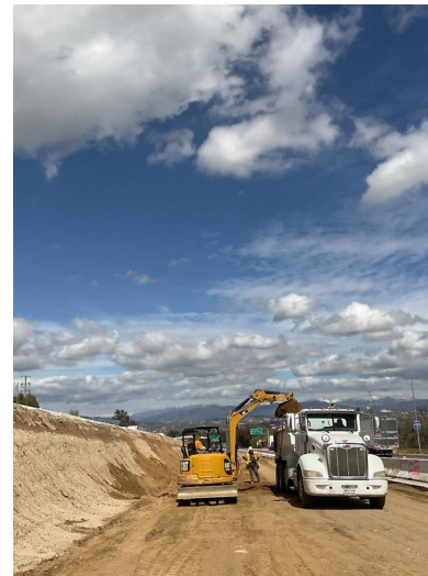
Structural Excavation for RW-2708
