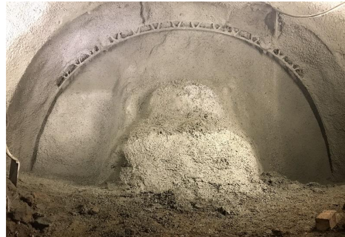
Cross Passage 35 excavation
