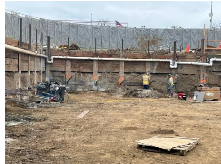
Westwood/VA Station: Tiebacks Installation– North & West Walls
