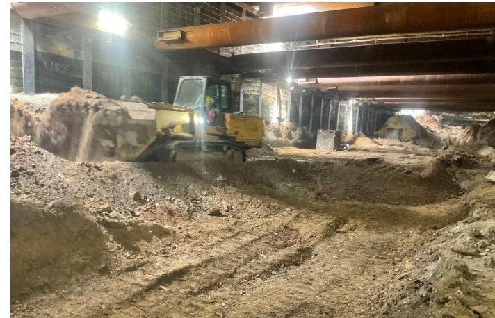
Westwood/UCLA Station: Excavation at Wilshire Blvd
