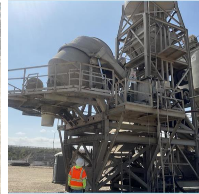
On-site concrete batch plant
