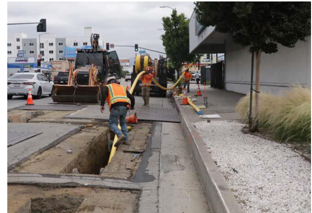
Installation of a 4" gas main by SCG on Van Nuys Blvd, just south of Saticoy.
