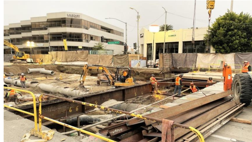
Wilshire/La Cienega Deck Removal/Street Restoration
