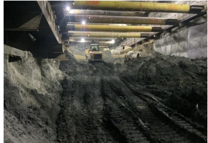
Century City Constellation Station - Excavation Progress
