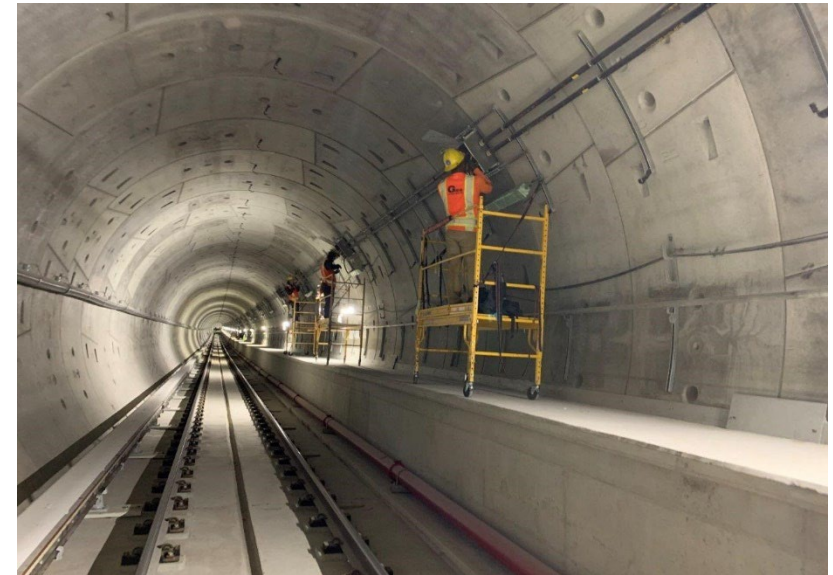
Reach 1 Tunnel Cable Installation
