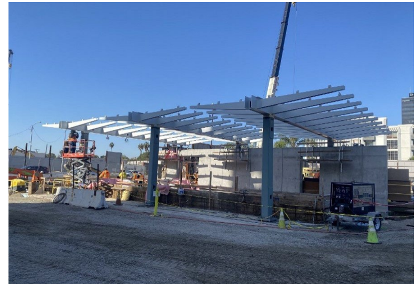
Wilshire/La Brea Station Canopy
