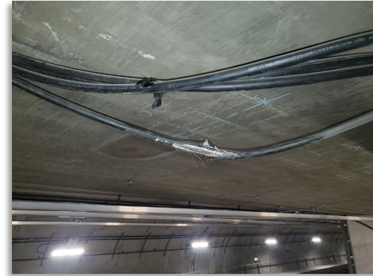
Failed feeder cable securement
