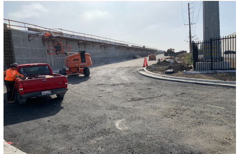
NB Crenshaw Blvd new on ramp to SB 405 (RW 799 and 803)
