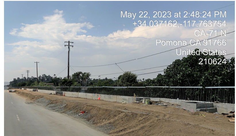
Retaining wall 161 and drainage system construction
