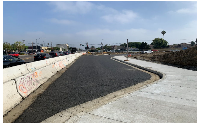
NB Crenshaw Blvd new loop ramp to NB 405
