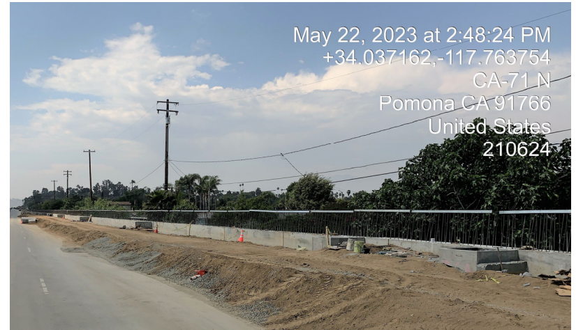
Retaining wall 161 and drainage system construction
