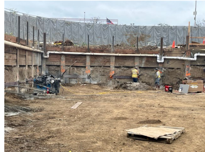
Westwood/VA Station: Tiebacks Installation– North & West Walls
