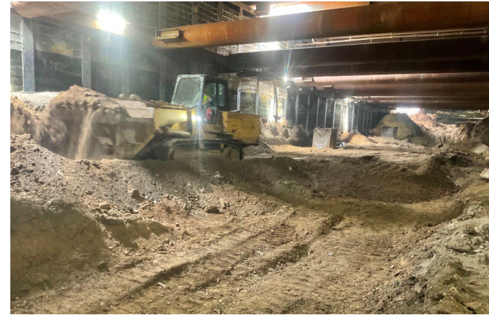
Westwood/UCLA Station: Excavation at Wilshire Blvd
