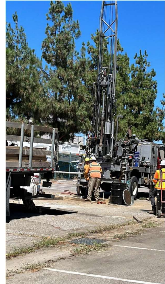
Geotech Investigations for Stormwater Capture
