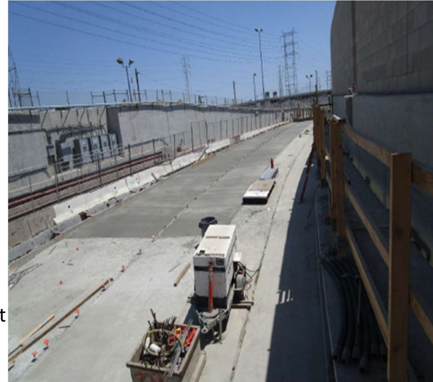
Portal –West Retaining Wall and invert
