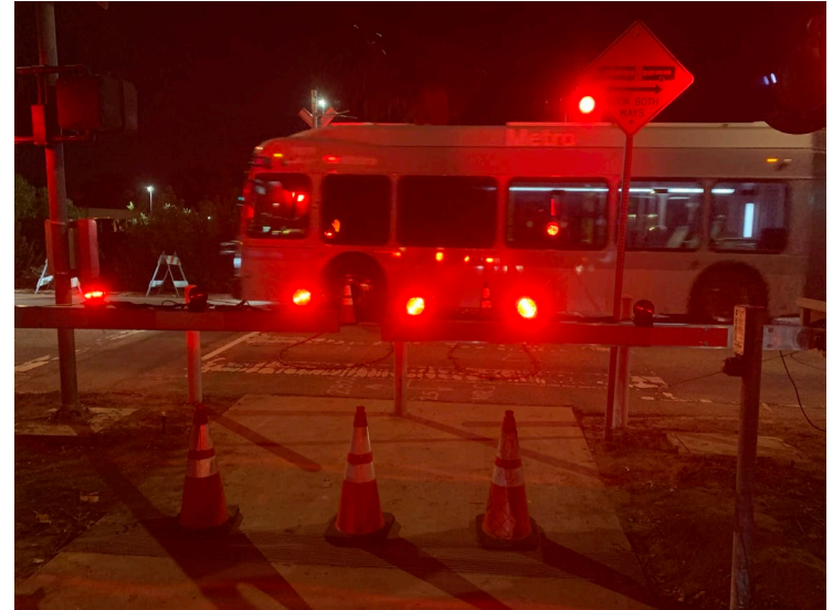
Pilot Gate - loop-based testing at Hayvenhurst
