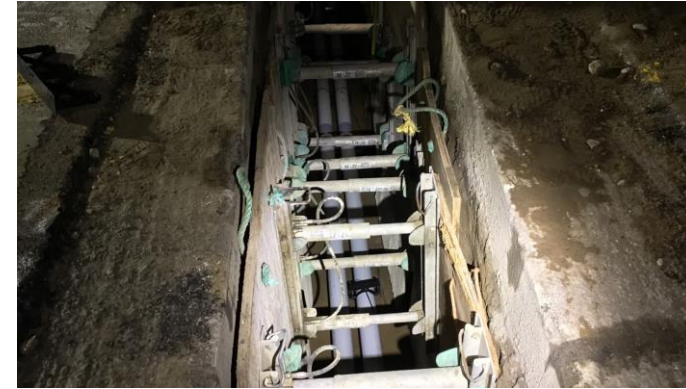
C1220 Ductbank Installation
