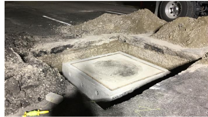
C1220 Manhole Installation
