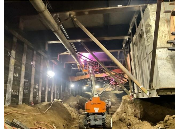
Westwood/UCLA Station: Welding of Transverse Bracing for Electrical Vault
