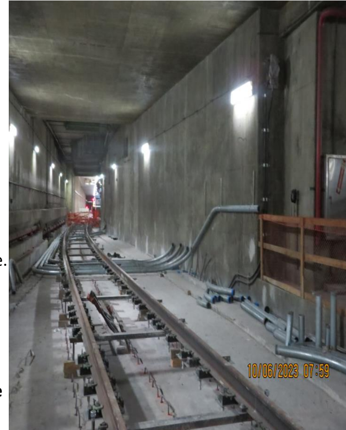
East Union Track Placement
