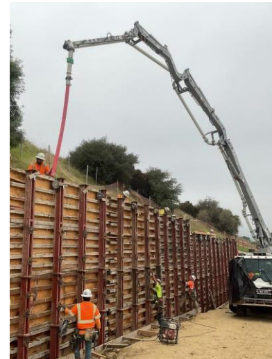
Pouring concrete at Retaining Wall 2461
