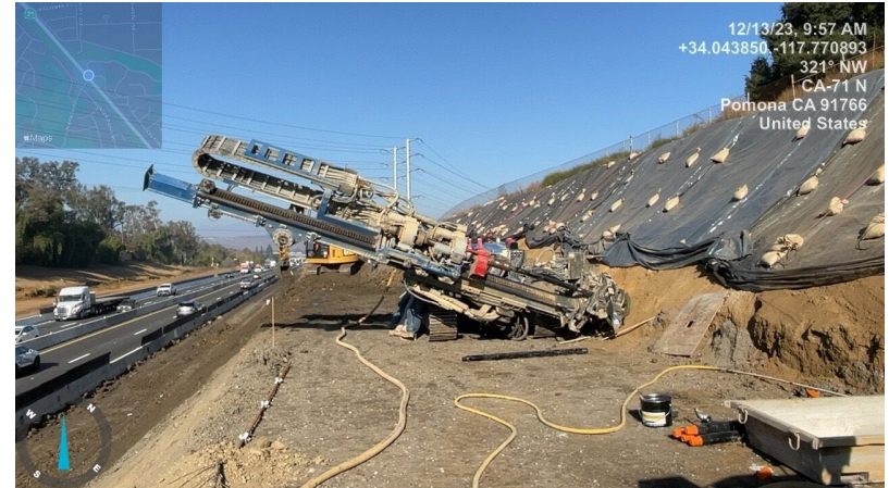
Retaining wall 131, verification soil nail drilling.
