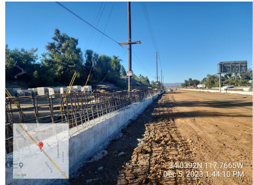
SR-71 SB, SW138 footing/wall.
