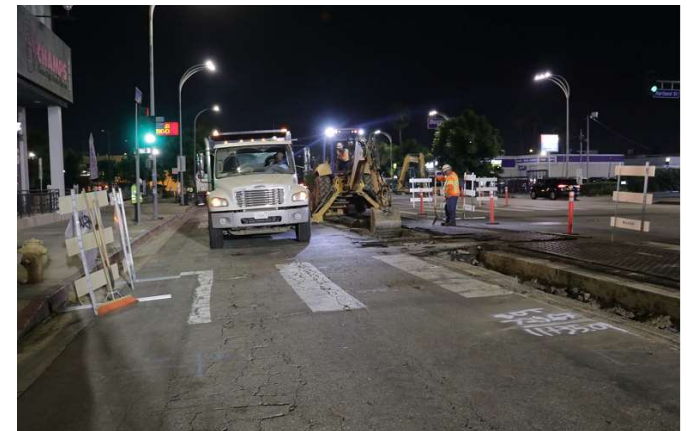
Duct bank installation in Van Nuys Blvd.
