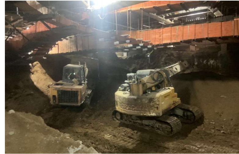
Westwood/UCLA Station: Excavation at Wilshire Blvd
