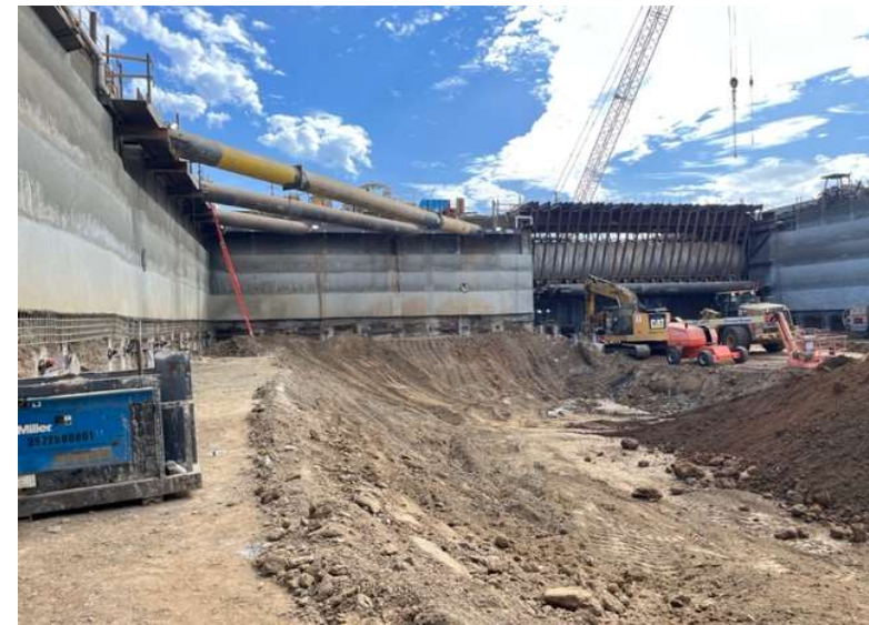
Westwood/VA Station: Tiebacks & Shotcrete Installation and Excavation
